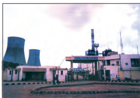
Fig 3.10: A view of a Thermal Power Station
