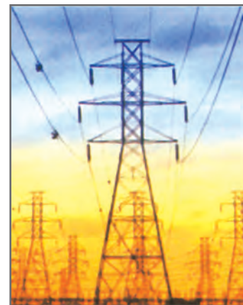
Fig. 3.7: National Power Grid to supply Electricity
